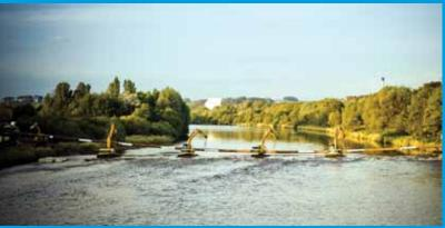
VolkerStevin completing the construction and installation of a 132m long, 609mm diameter pipeline during low tide across the River Lune, Lancaster.
