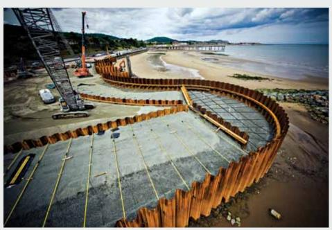
Installation of piling and tie rods at Colwyn Bay
