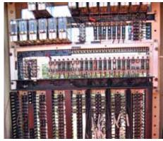
New wires run in existing location case ready for terminating during commissioning stage
